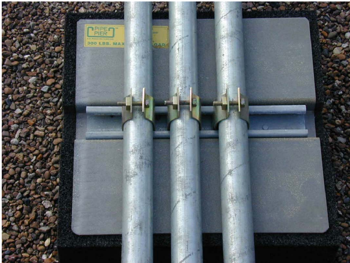
05 ROOF MOUNTED RACEWAY SUPPORT DETAIL
