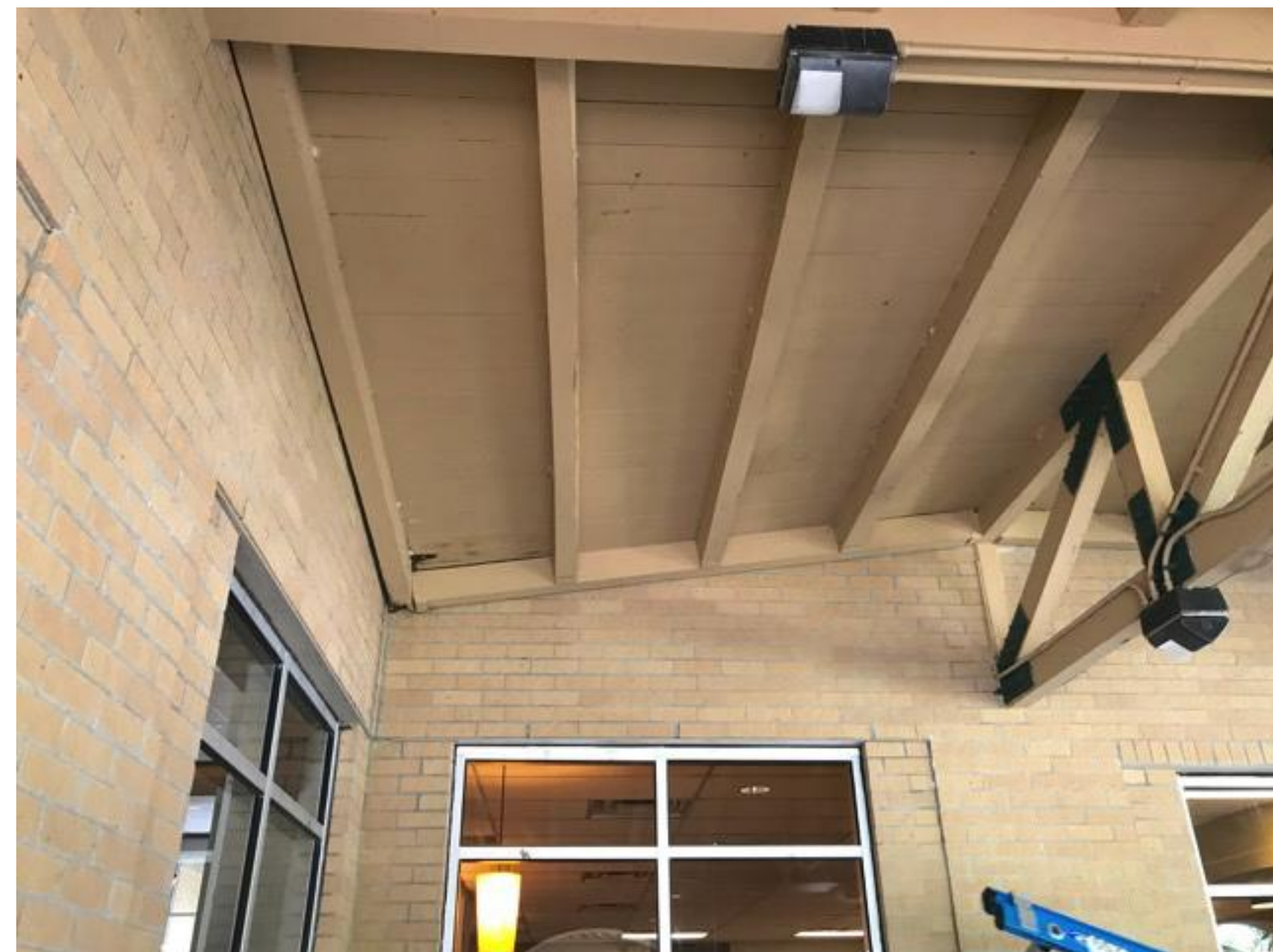
PHOTO OF EXISTING CONDITION
