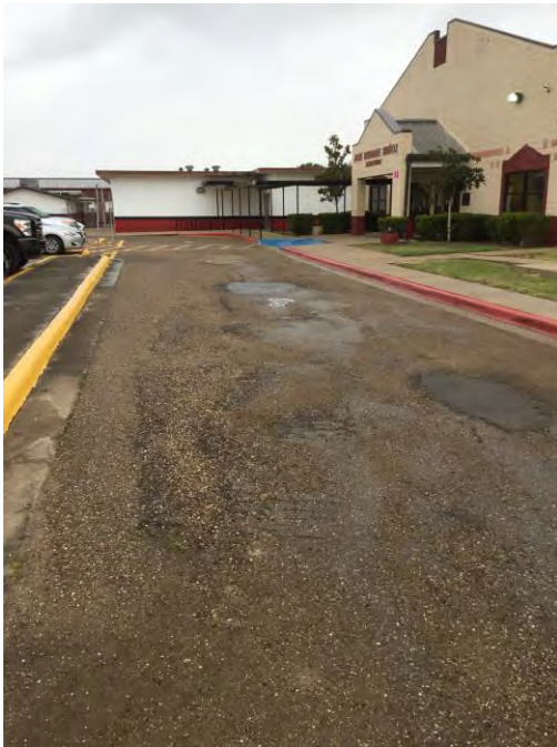
Photographs 3 and 4: Pavement Distresses Within the Existing Driveways of the La Villa ISD J. B. Muñoz E.S. Campus
