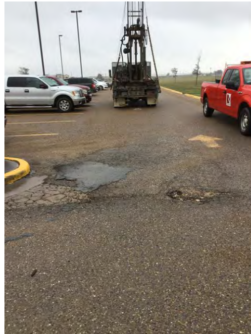
Photographs 3 and 4: Pavement Distresses Within the Existing Driveways of the La Villa ISD J. B. Muñoz E.S. Campus
