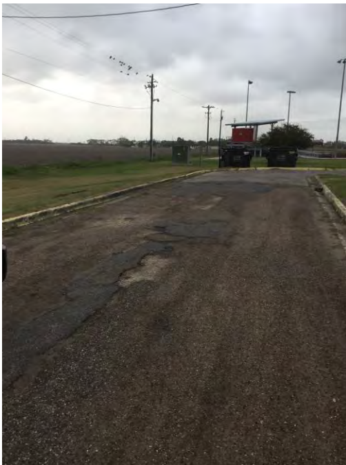
Photographs 1 and 2: Pavement Distresses Within the Existing Driveways of the La Villa ISD High School Campus
