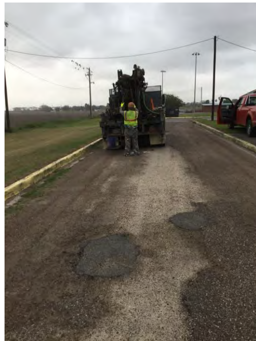
Photographs 1 and 2: Pavement Distresses Within the Existing Driveways of the La Villa ISD High School Campus
